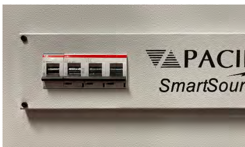
Figure 5-3: Mains CB in OFF (lower) Position
